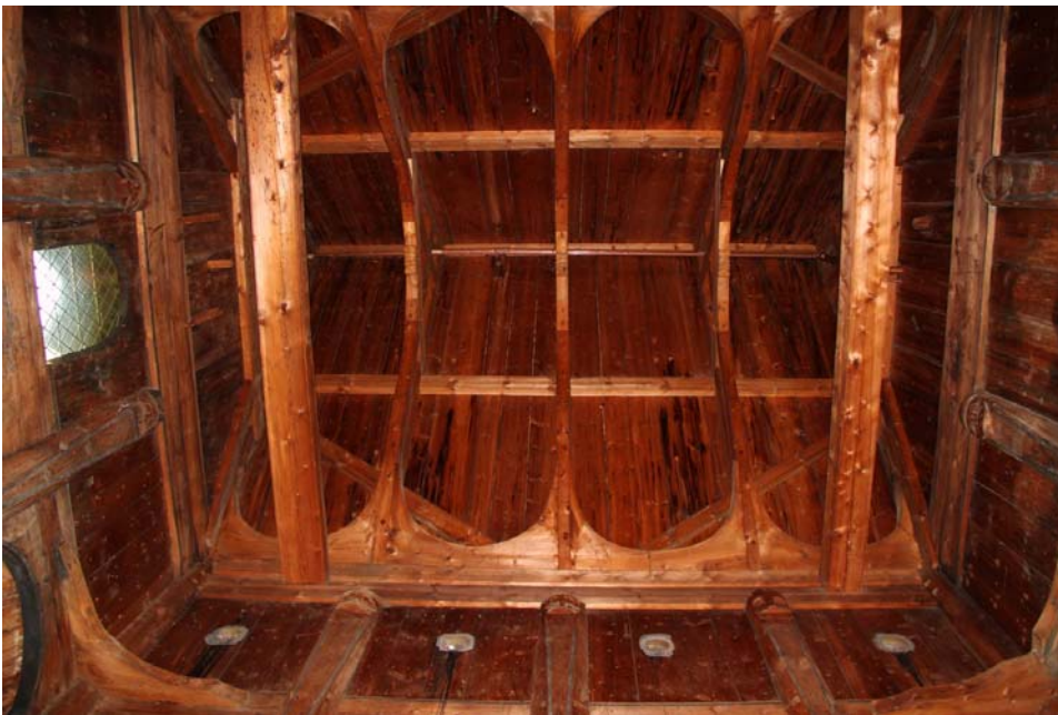
Fig. 10 – The roof support in the Borgund stavkirke . The ledges are those curved shapes that link the struts of the truss and fix them at the bottom. The curved shape is obtained by joining two ledges. The masks decorating the end of the posts or stav can be seen, as in fig. 4.
